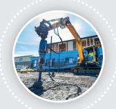
STEP 4 Install your screw piles to required torque measurement.
